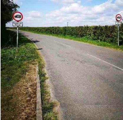
Figure 2-5: High Ditch Road- Site Visit
